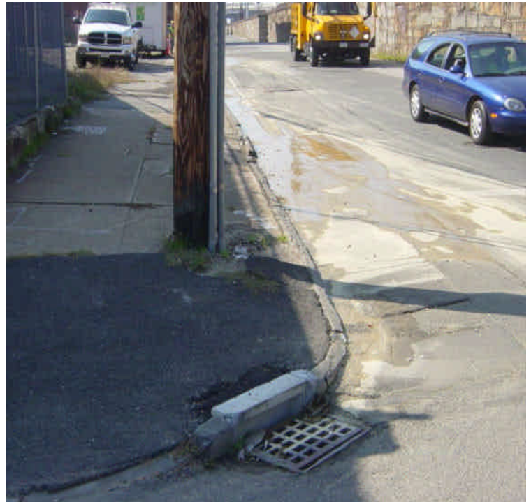
Silt and runoff were observed along the roadway near sta. #790 which was attributed to the ongoing vault work. A downgradient catch basin was not protected. Runoff or dewatering from future vault work activities should be contained and catch basins should be protected to prevent sedimentation.
