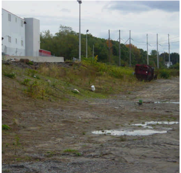
The exposed soil along the slope near sta. #1080 has re-vegetated naturally (approximately 50% coverage). The slope will be fully restored in the future. A plan is being worked out with the landowner.
