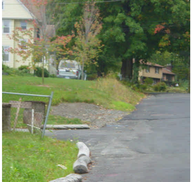
Exposed soil on the slope near sta. #1049 (vault #3) remain temporarily stabilized and contained with hard-pack and barrier controls.
