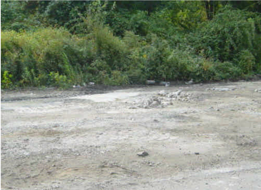
Concrete washouts continue to be observed near sta. #1017. M/N contractors are not currently working in this area and have stated that the washouts are not from project related activities and are the result of other construction in the area.
