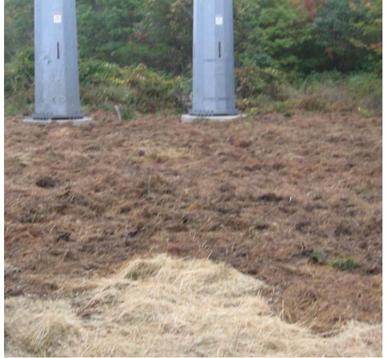
West River St: Restoration efforts are complete at structure #3836.
