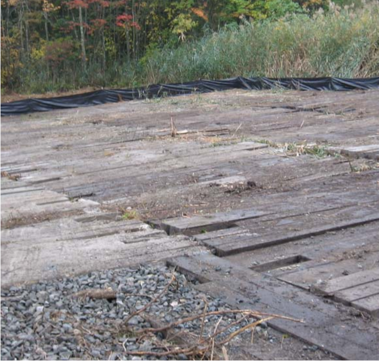
West River St (Milford): Pad Reclamation is complete at proposed structure #24023. Controls are in place.
