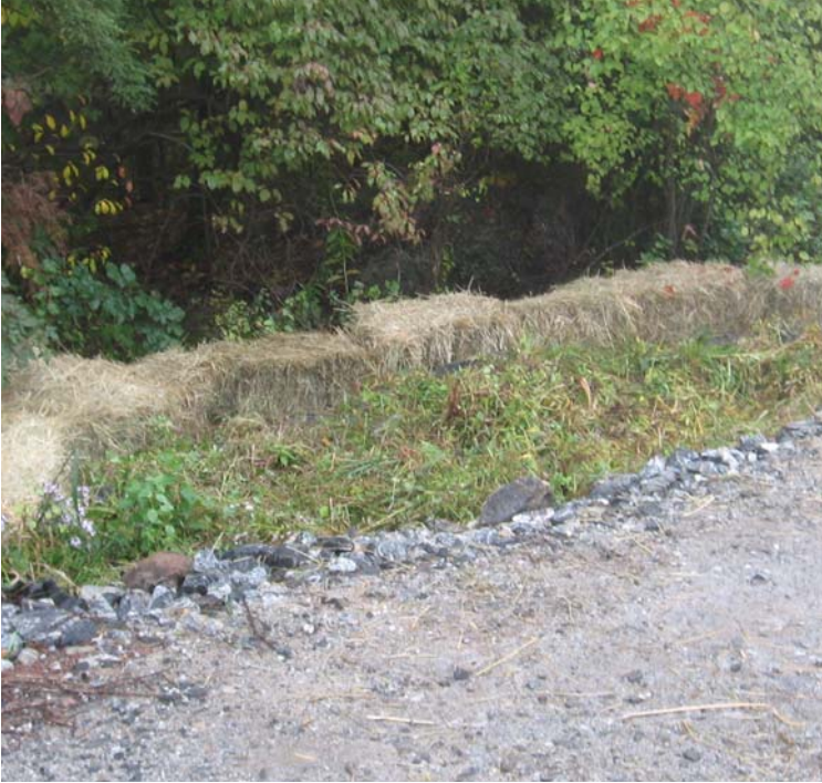
Gaylord Mtn Rd (Hamden): Sediment has been removed from the stone trap and a new line of haybales was installed.
