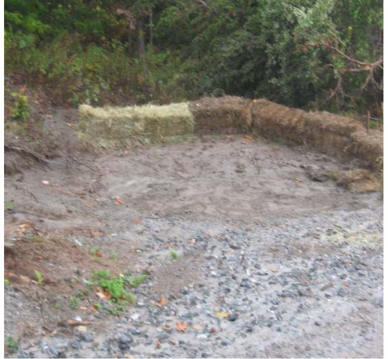
Brooksvale Ave (Hamden): Sediment has been removed from the sediment trap and the haybale line has been extended here.
