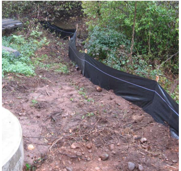
Willow St (Hamden): Silt fence has been installed along Willow Brook.
