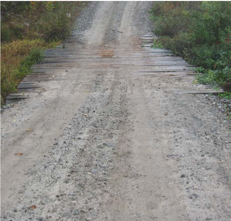
Brooksvale Ave (Hamden): A view of the wetland crossing at wetland #100. Sediment migration from the access road is not an issue at this crossing.
