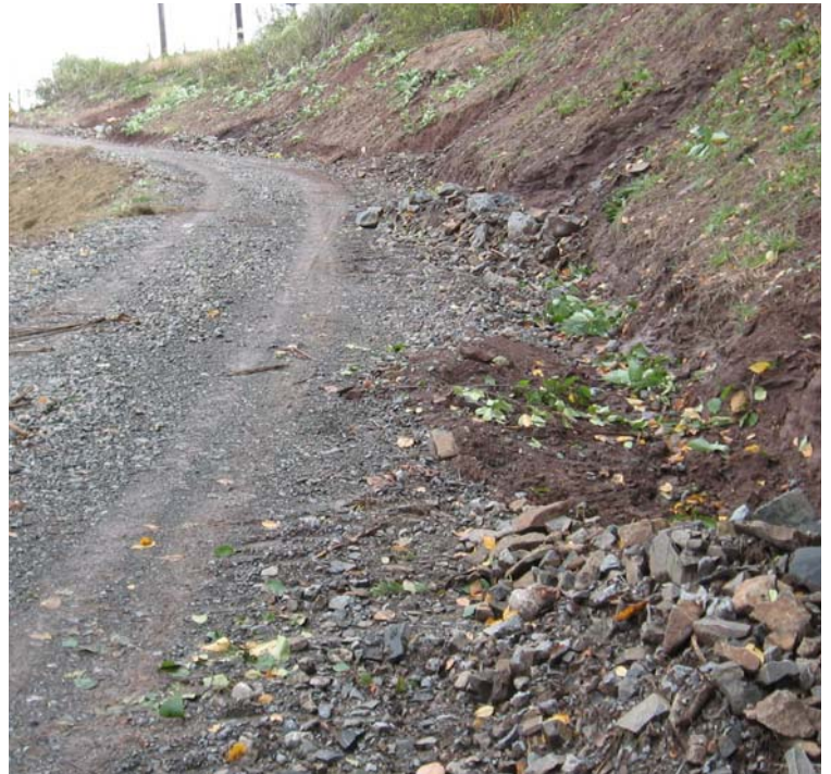
Old Lane Rd: Additional view of the stone check dams.
