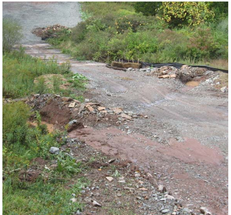
Old Lane Rd: Additional controls have been installed upgradient of wetland #94.
