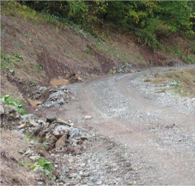
Old Lane Rd: Several modified stone check dams have been installed along the access road here.
