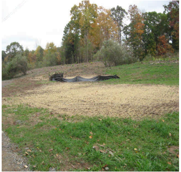
Durham Rd: Exposed soils were graded and seeded.
