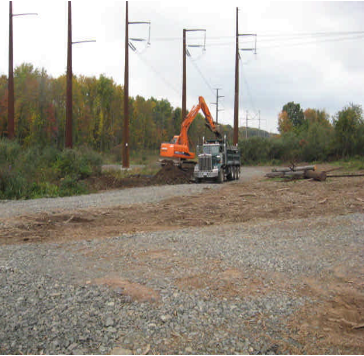
Carpenter Ln: Crews were removing soil stockpiles.
