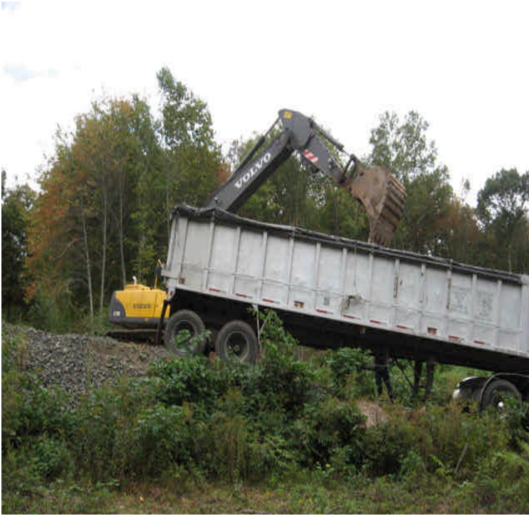
High Hill Rd: Crews were removing soil stockpiles.
