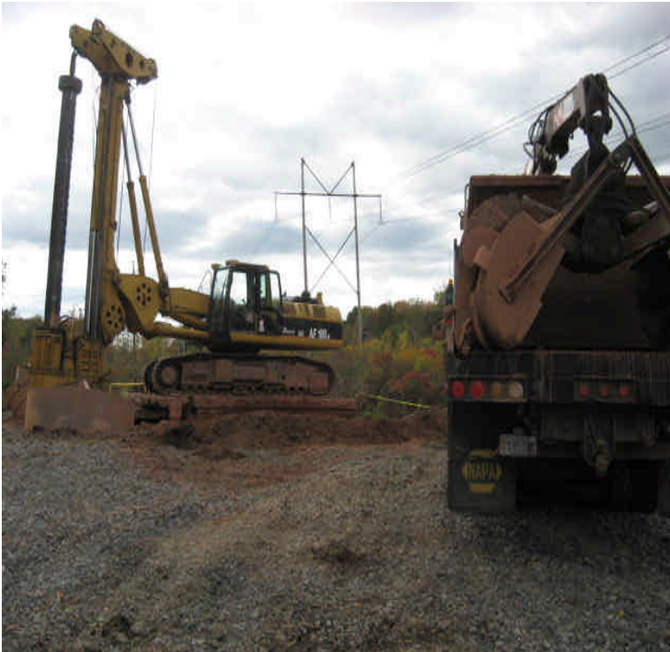
Tamarack Swamp Rd: Foundation drilling in the wetlands continues.
