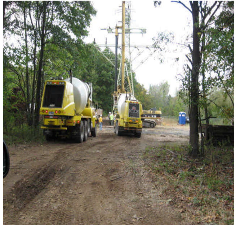
Pent Rd: Foundation drilling continues.
