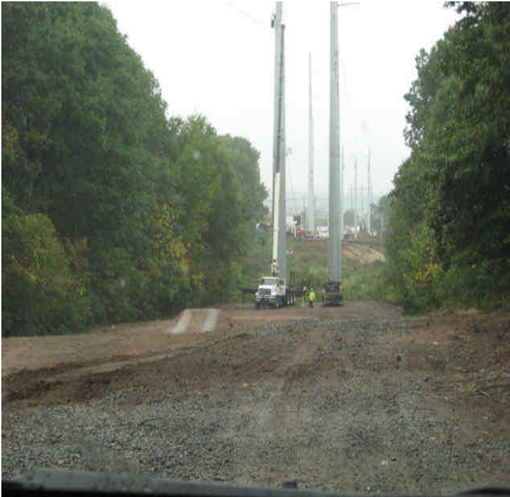
Docker Dr: Exposed soils remain graded, mulched, and seeded. Crews were performing line work.
