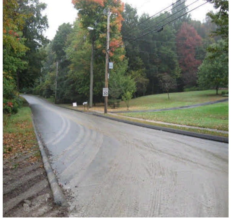
High Hill Rd: Some sediment tracking was noted on the roadway.
