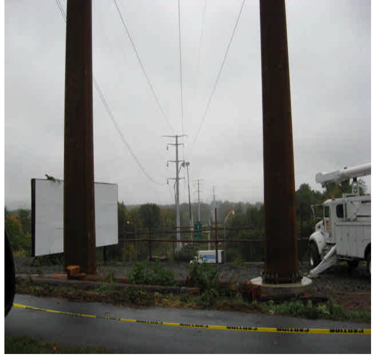
I- 91: Crews were pulling lines across Route 91 to Docker Dr.
