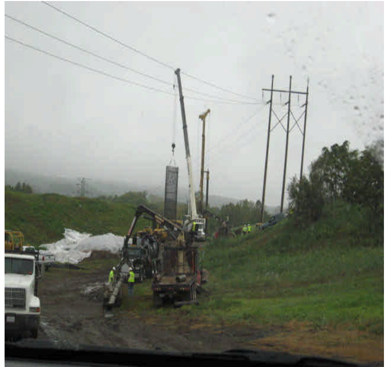
Pent Rd: Foundation installation was underway.
