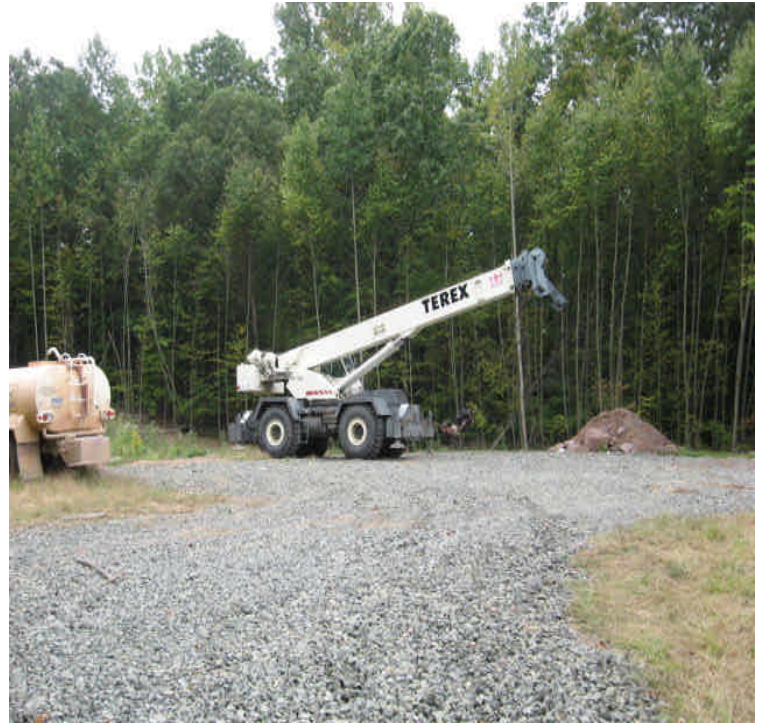
Tuttle Ave: Pole installation equipment was being stored here.
