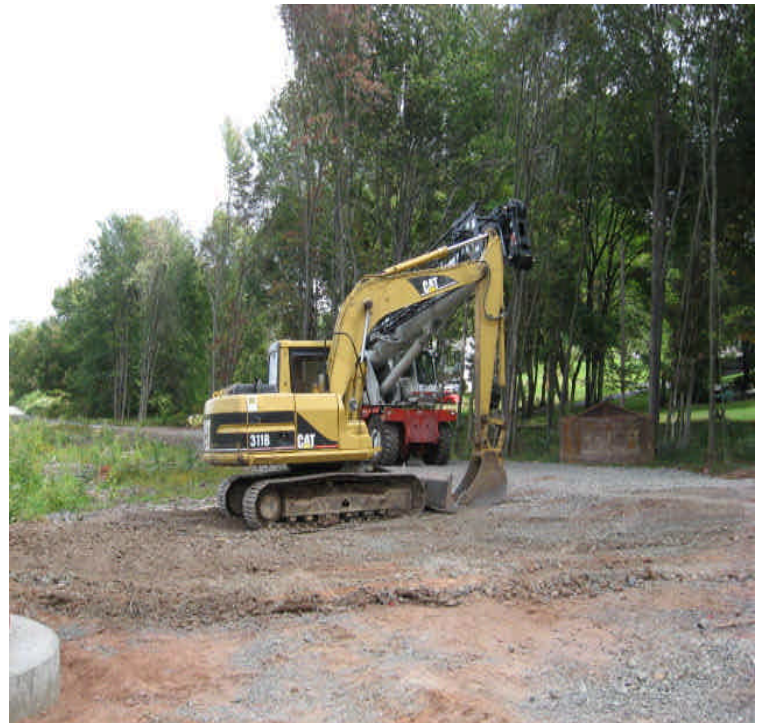
Powers Rd: Restoration efforts adjacent to wetlands are complete for now.
