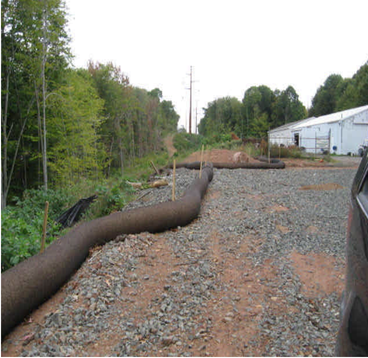
Harrison Rd: Fiber sock installed along the pad site and stockpile.
