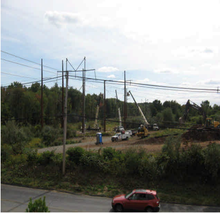
Carpenter Ln: Line work is underway.
