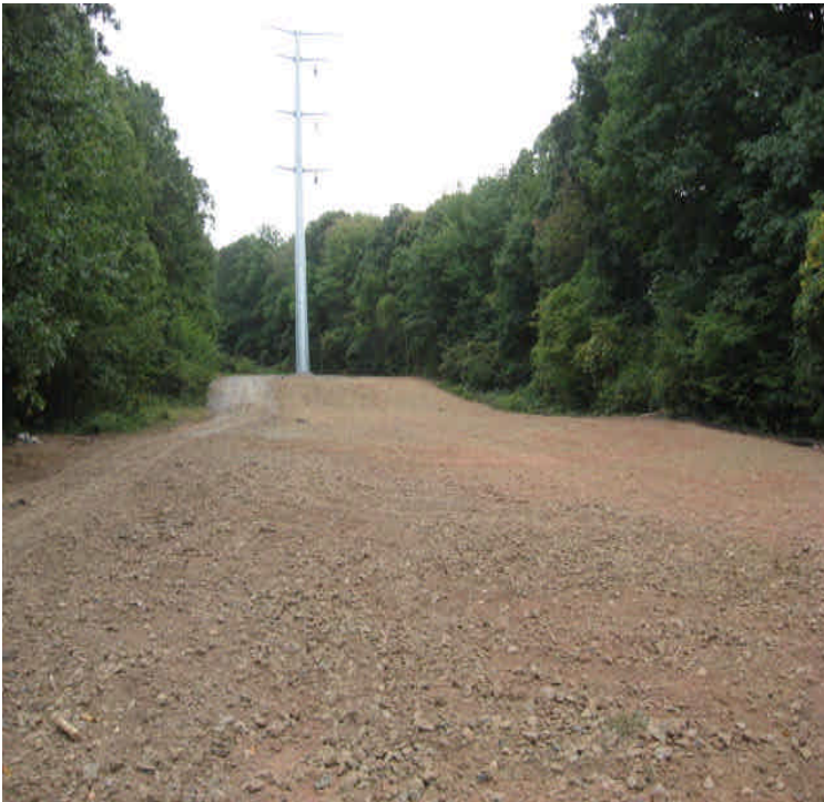
Docker Dr: Exposed soils have been graded, mulched, and seeded.
