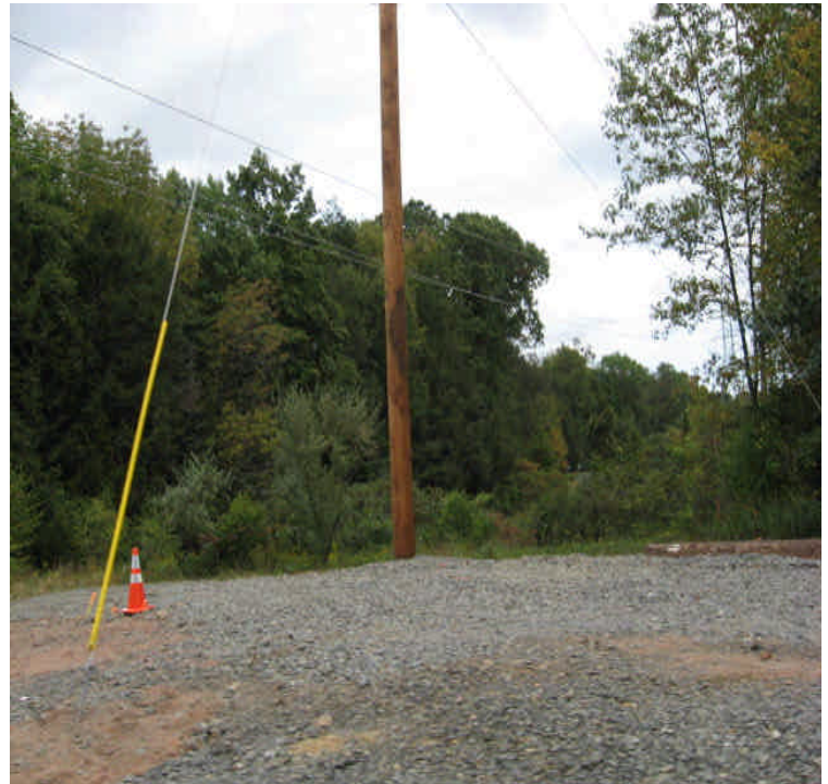
Old Farms Rd: New poles were installed along the ROW.
