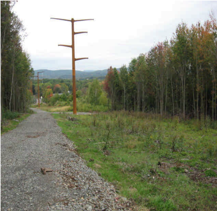
Vegetative cover has established on the seeded portion of the ROW and the area is stable.
