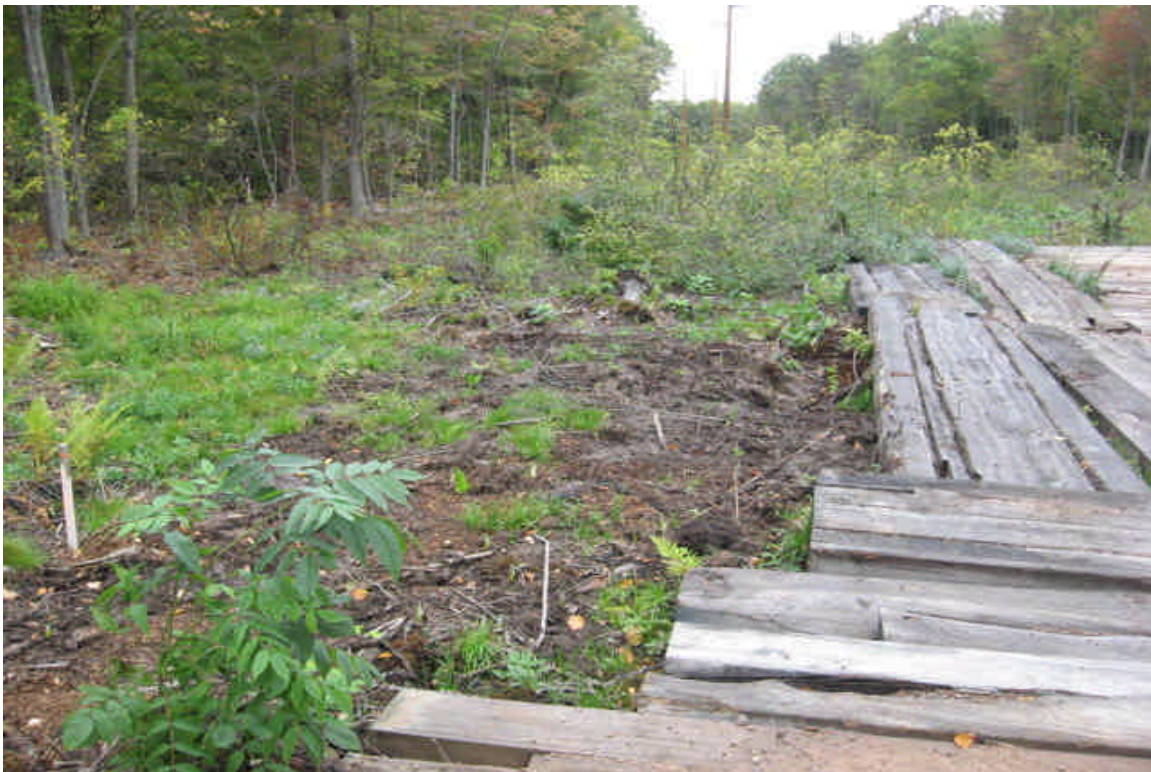
Equipment ruts have been filled in and soils have been regraded. Monitor for stabilization.
