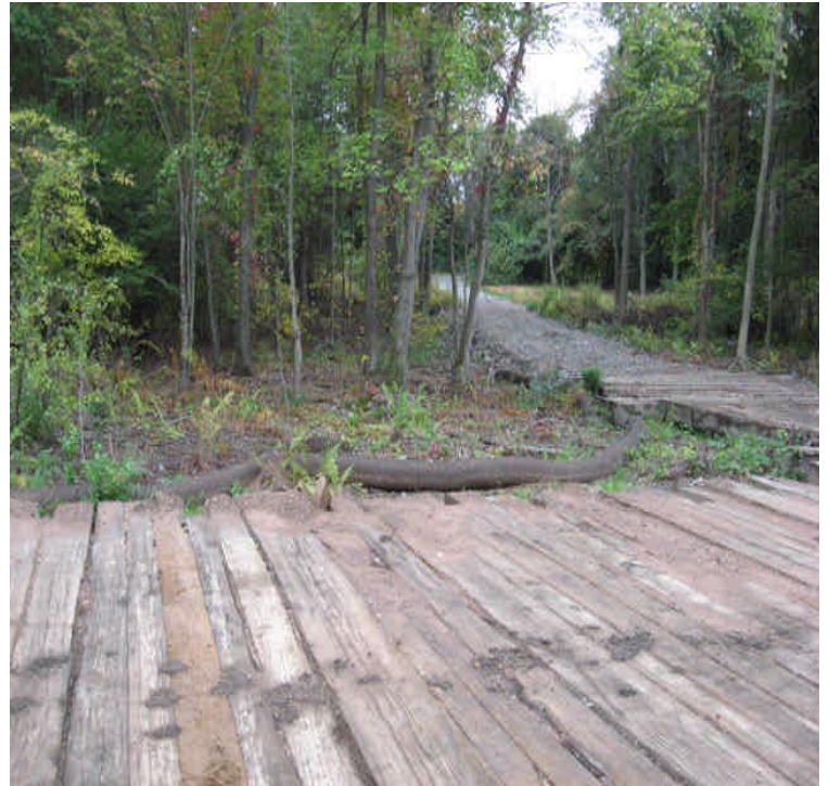
Sediment was removed from mats and wetlands. Controls are in place
