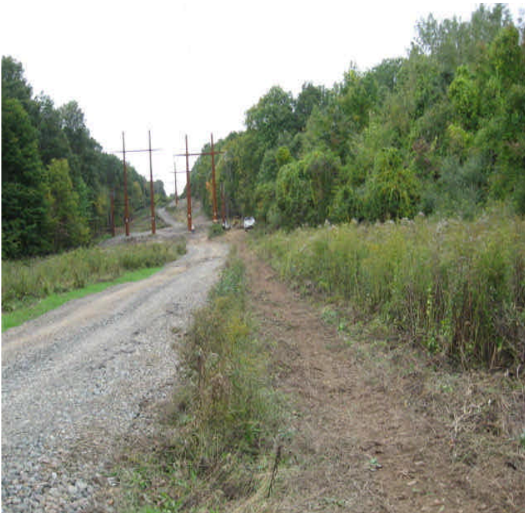
Black Walnut Dr: Crews were installing grounding wires.
