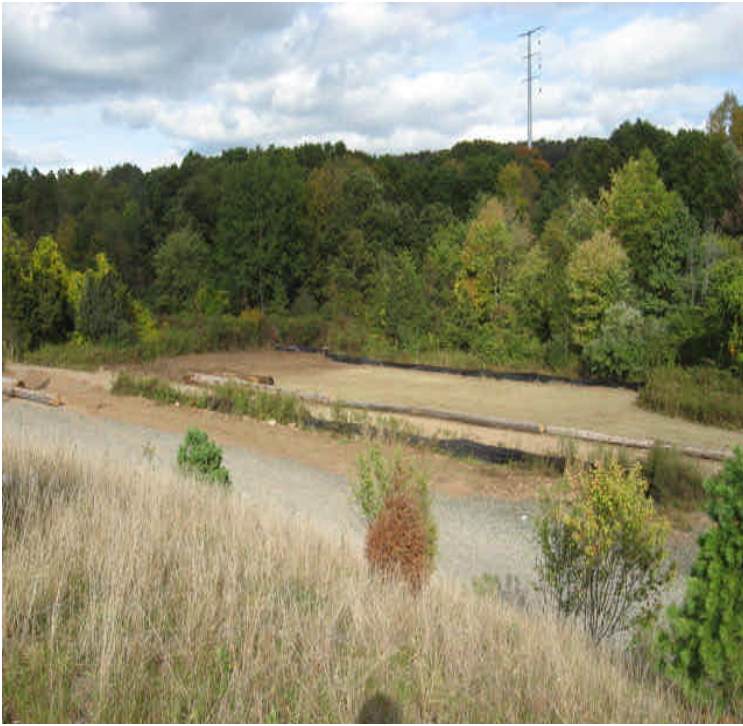
Beseck SS: The original ROW access off Carpenter Ln. was upgraded and is now in use. The constructed access between Beseck and the ROW remains blocked off. Adjacent disturbed areas were graded and seeded.
