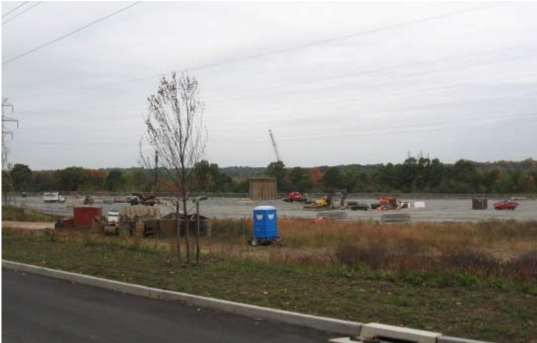
A view of the foundation work at the East Devon Substation.
