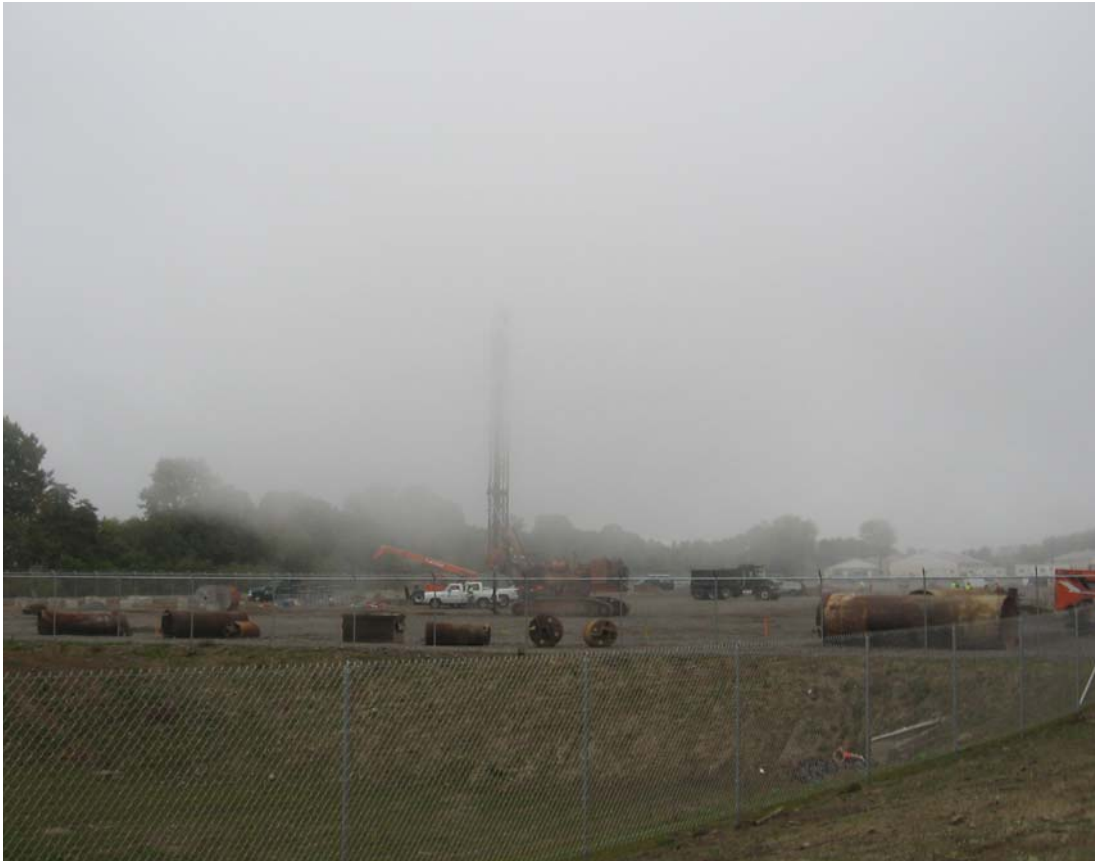
A view of the foundation work at the East Devon Substation.
