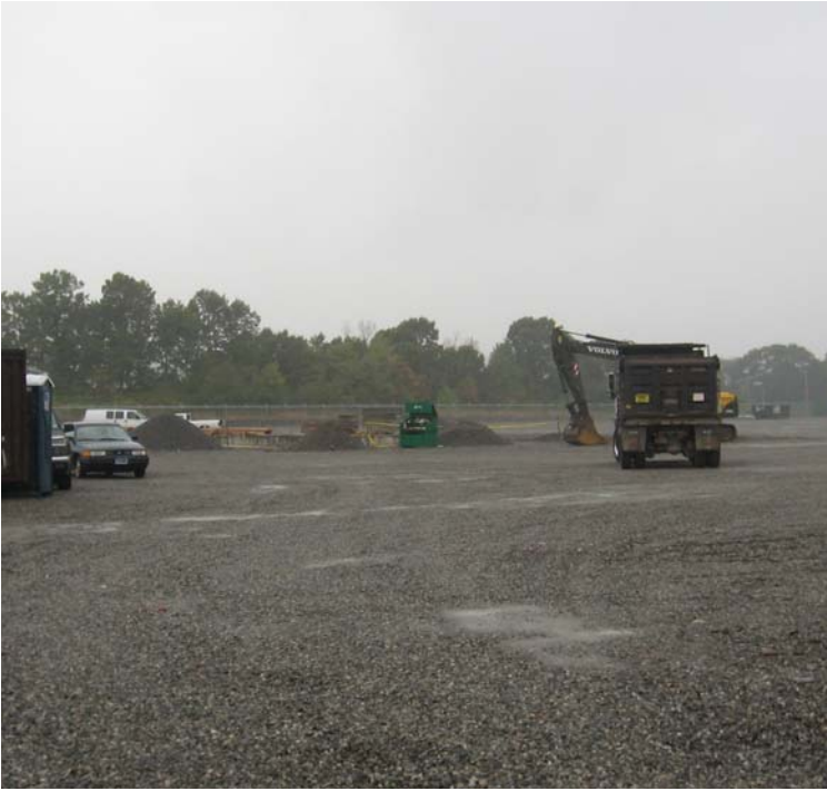
Foundation work continues here this week.
