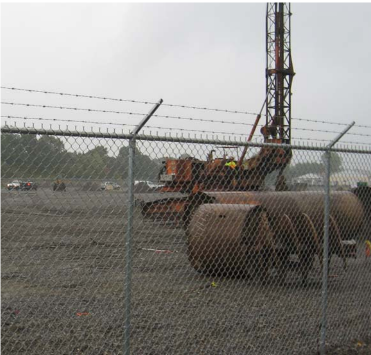
Foundation drilling was observed within the yard this week.
