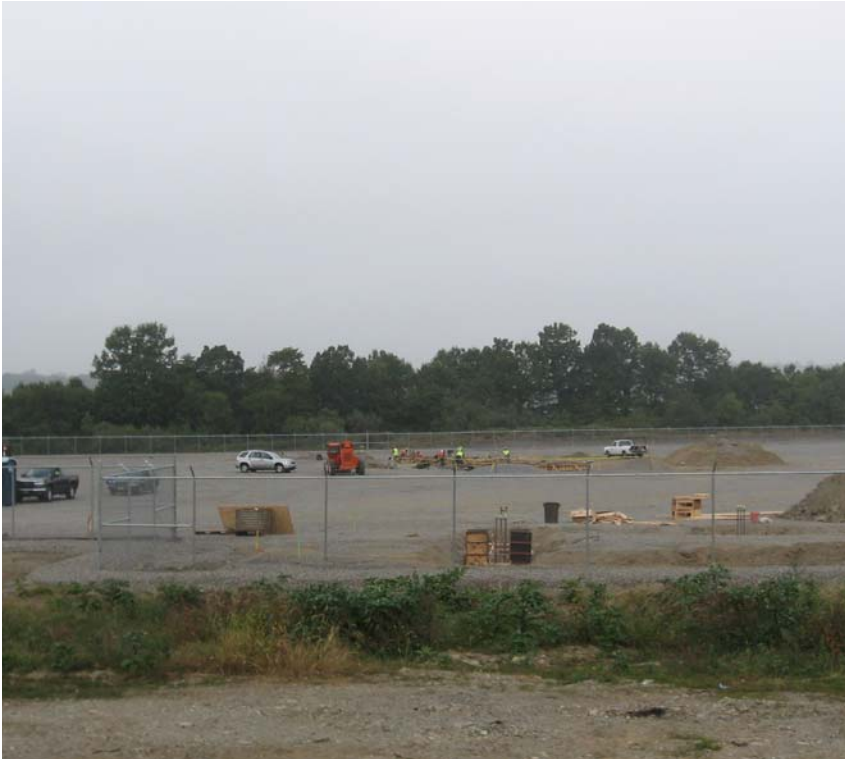
Foundation work continues at the East Devon Substation.
