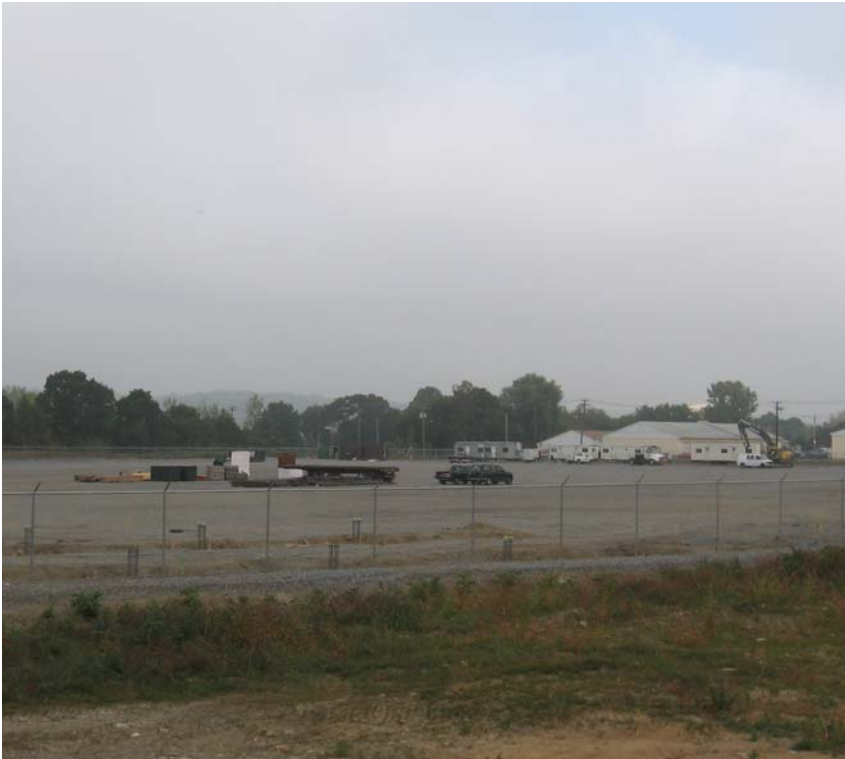
Additional view of the East Devon Substation.
