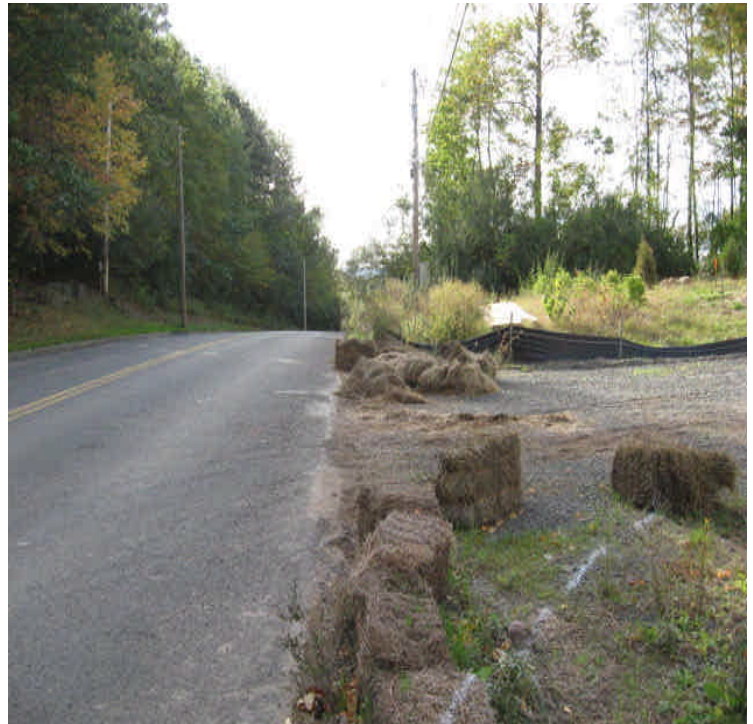
Haybales were removed from the western site entrance.
