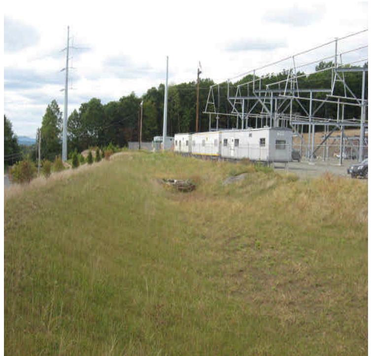
View of the stabilized detention basin onsite.
