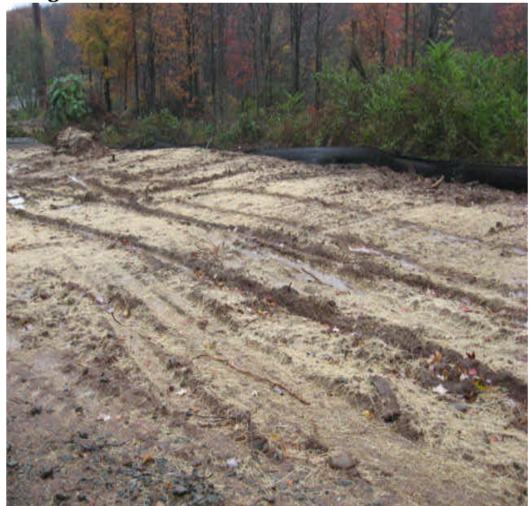
Woodhouse Ave: The stockpile was removed and the area remains mulched and seeded. Controls are in place and working well.
