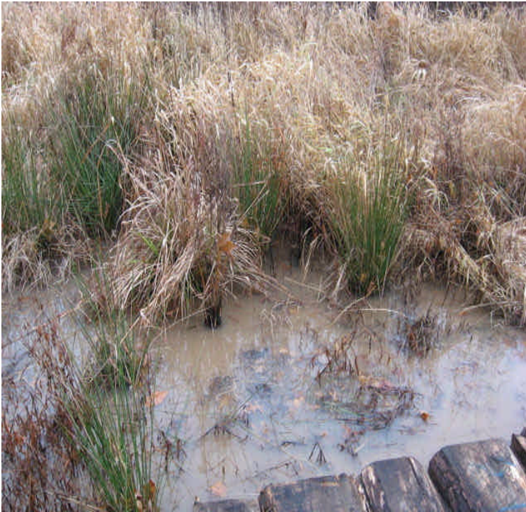
Durham Rd Golf Course: Turbid water was flowing into wetlands from the access road.
