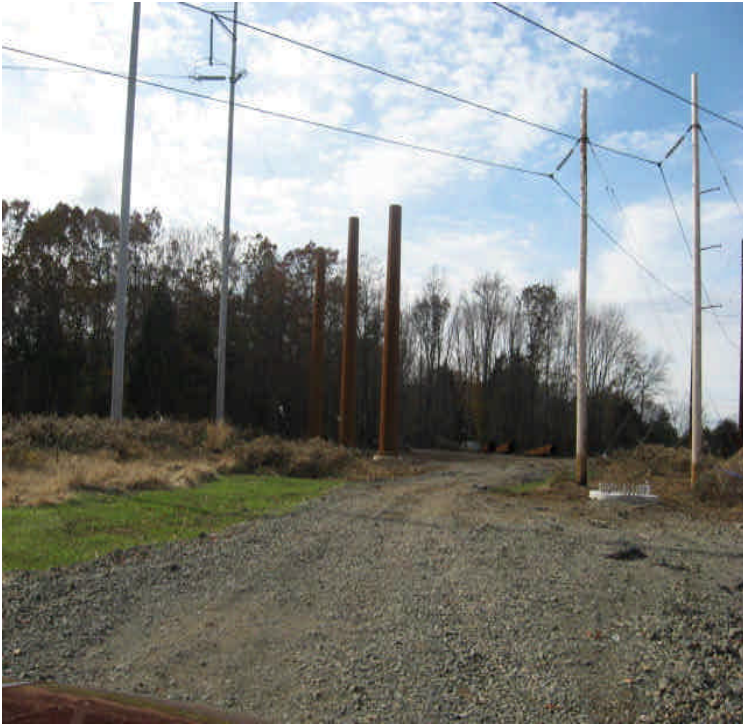
Oxbow Jct: Partially completed structures waiting for final line transfer.
