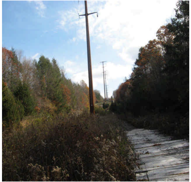
Haddam Quarter Rd: Timber mat crossing. Vegetated cover has established and stabilized the adjacent wetlands.
