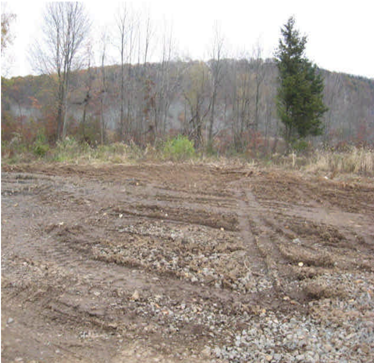
South of East Main St: (Both photos) Large, disturbed soil area located upgradient from wetlands. Controls are needed here. Grade, remove stone, and temporarily stabilize the soils if work will not return in 21 days.
