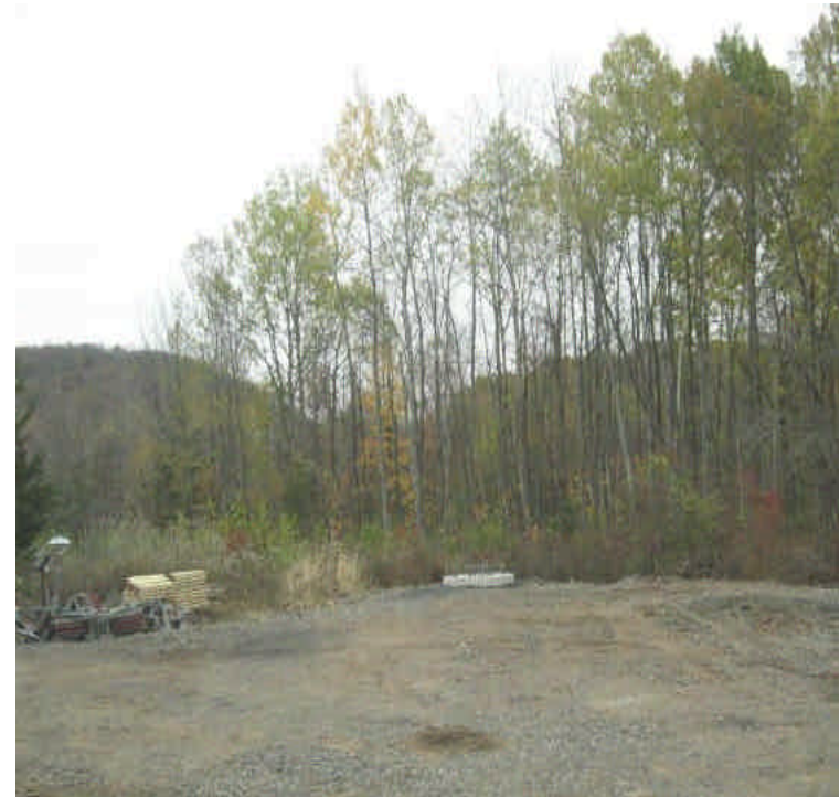
South of East Main St: (Both photos) Large, disturbed soil area located upgradient from wetlands. Controls are needed here. Grade, remove stone, and temporarily stabilize the soils if work will not return in 21 days.
