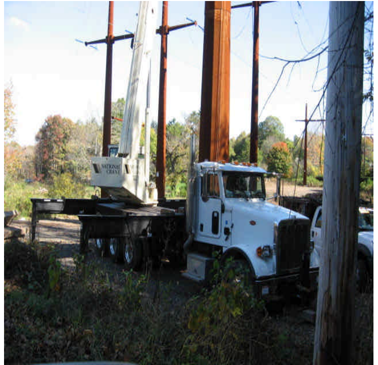
Oxbow Jct: Line work underway. Area is stable.
