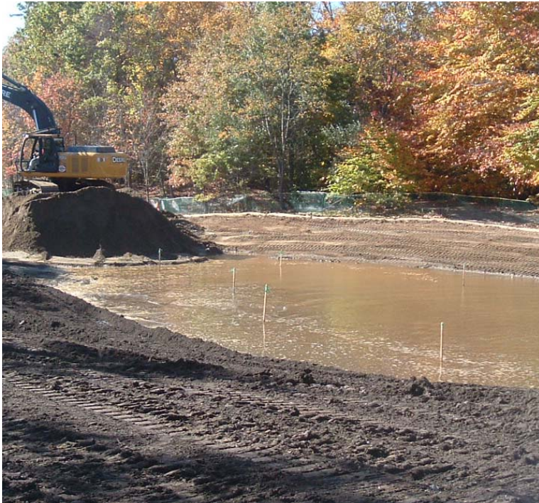
Eisenhower Park (Milford): Construction of the wetland mitigation area continues.
