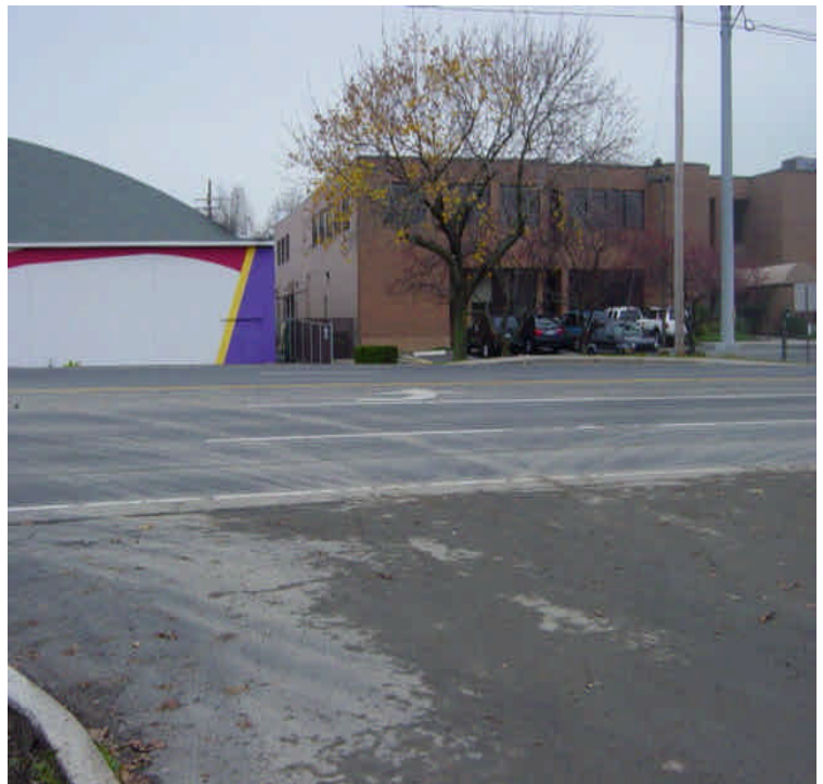
Entrance to the Kings Highway Laydown Yard. Some minor sediment tracking from the yard was noted on the roadway. This yard is also covered by the 4a report.
