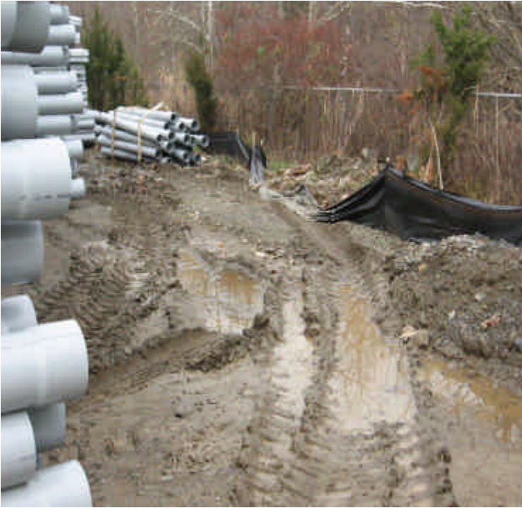
Both photos show areas along the perimeter silt fence which are in need of repair. This is along the edge of the yard adjacent to the sensitive areas.
