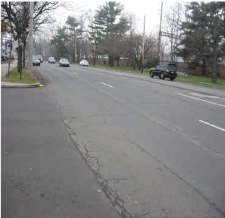
Trenching activities along Rt. 1 near its intersection with Mill Plain Rd.
