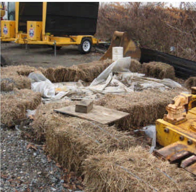
Attachment containment area in western side of the yard is not fully enclosed with controls.
