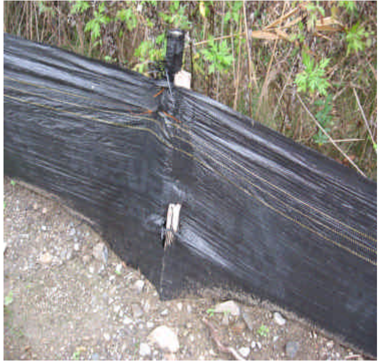
Both photos show areas along the perimeter silt fence which are in need of repair. This is along the edge of the yard adjacent to the sensitive areas.
