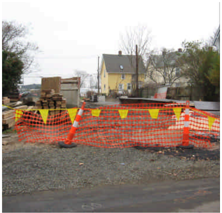
Photo of trenching activities located between Broad St. and Main St.
