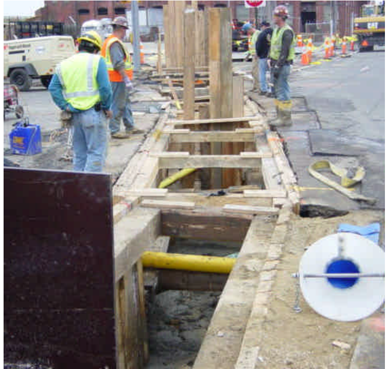
Trenching activities at the intersection of Railroad Ave. and Bostwick Ave.
