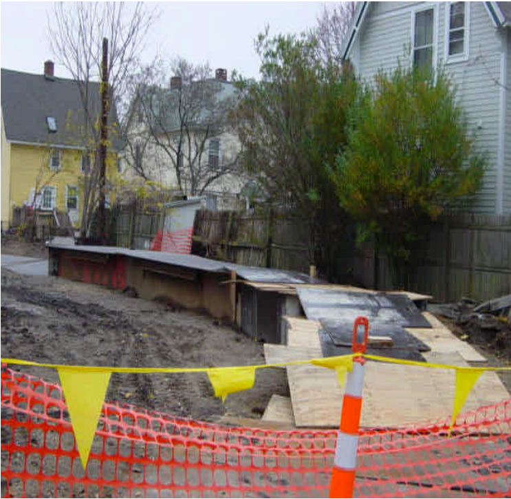
Photo of trenching activities between Broad St. and Main Ave.
