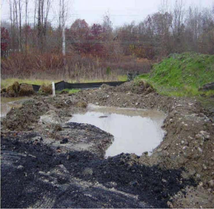
Both photos are of the former concrete washout basin and sweeper washout area in the Kings Highway Laydown Yard. The concrete basin has been removed and the sweeper washout area remains, (shown to the left). Continue to effectively contain the run-off to the yard.
