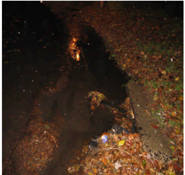
Photo of the catch basin located on Old Post Rd. that receives stormwater from the Fairfield Inn area. Please note that the runoff flowing into the catch basin contains no observable sediment.
