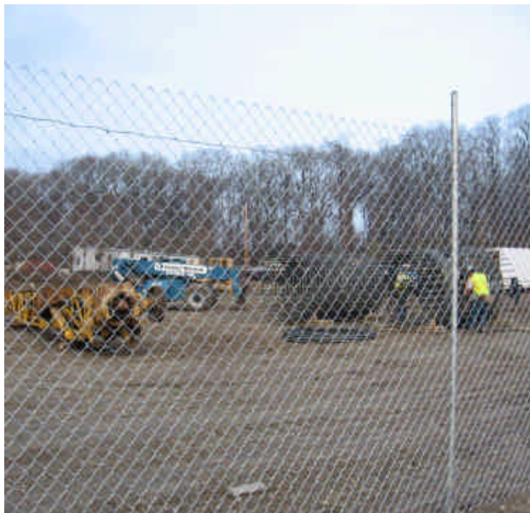
View of the contractor yard located off Shelland Street in Milford.
