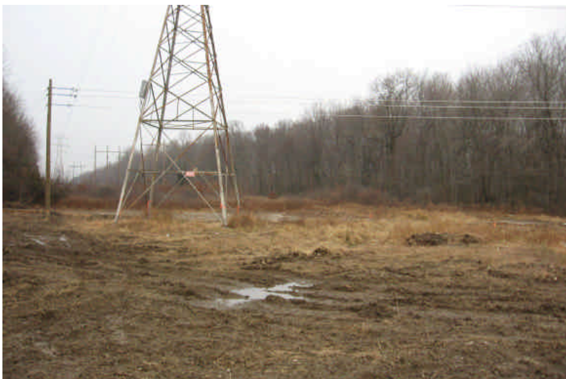
View of the matted (non-federally jurisdictional) wetland area in the ROW off Pease Road in Woodbridge. Major clearing will be necessary in the future for the relocation of the ROW here.
