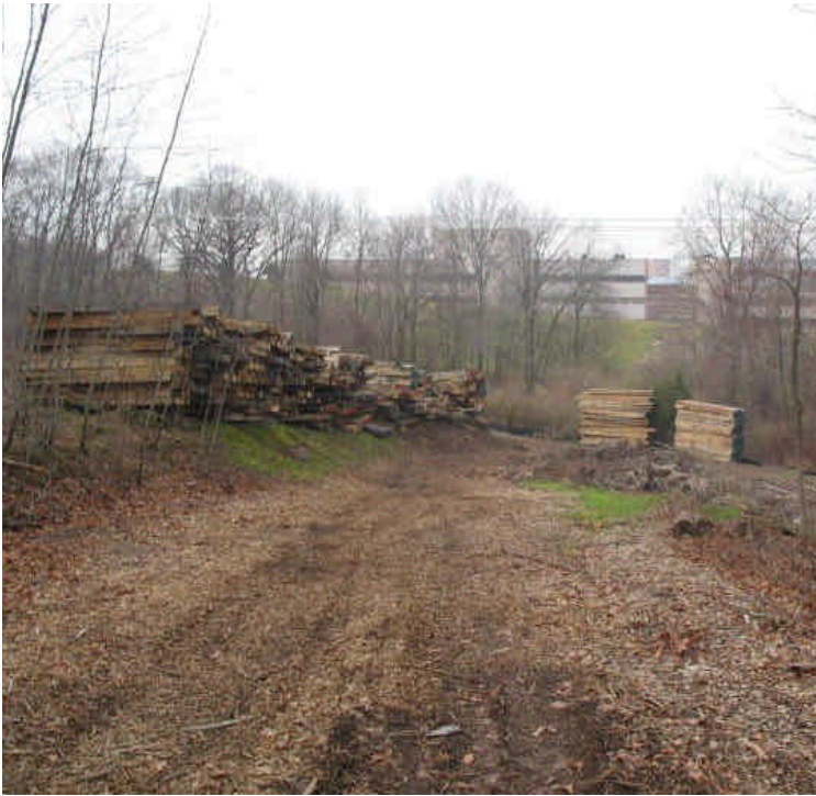
Wetland crossing/timber mats stored off High Hill Rd.
