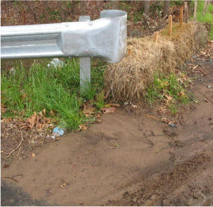
Sediment accumulation should be removed from the haybales at the ROW entrance off Mansion Rd.
