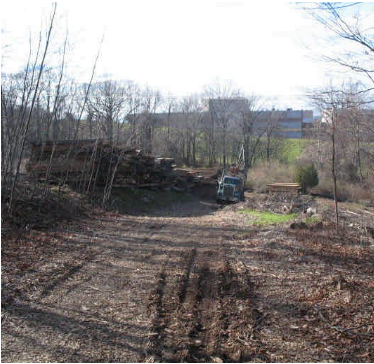
Wetland crossing mats stored off High Hill Rd.
