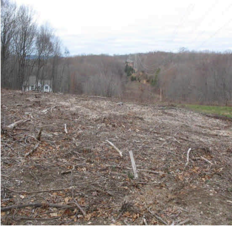
View of clearing previously completed off Mansion Rd.
