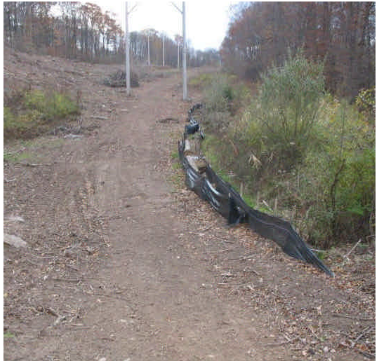
Silt fence above wetland off High Hill Rd.
