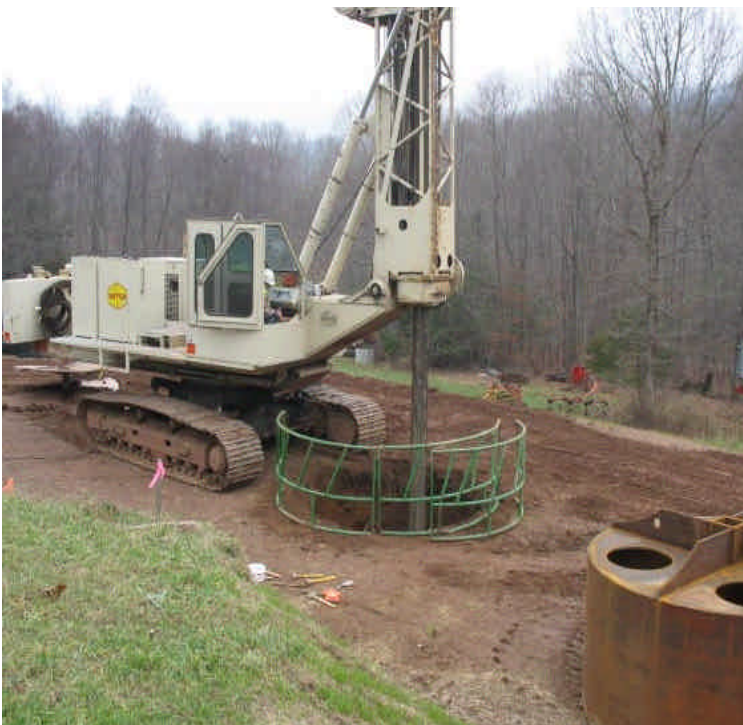
Foundation drilling north of Beseck SS.
