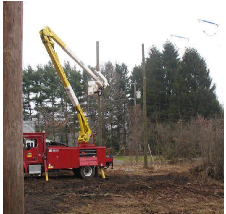
Pole installation and line work off Little Lane.
