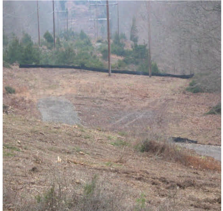
Silt fence, clearing and grading off Arbutus Street.
