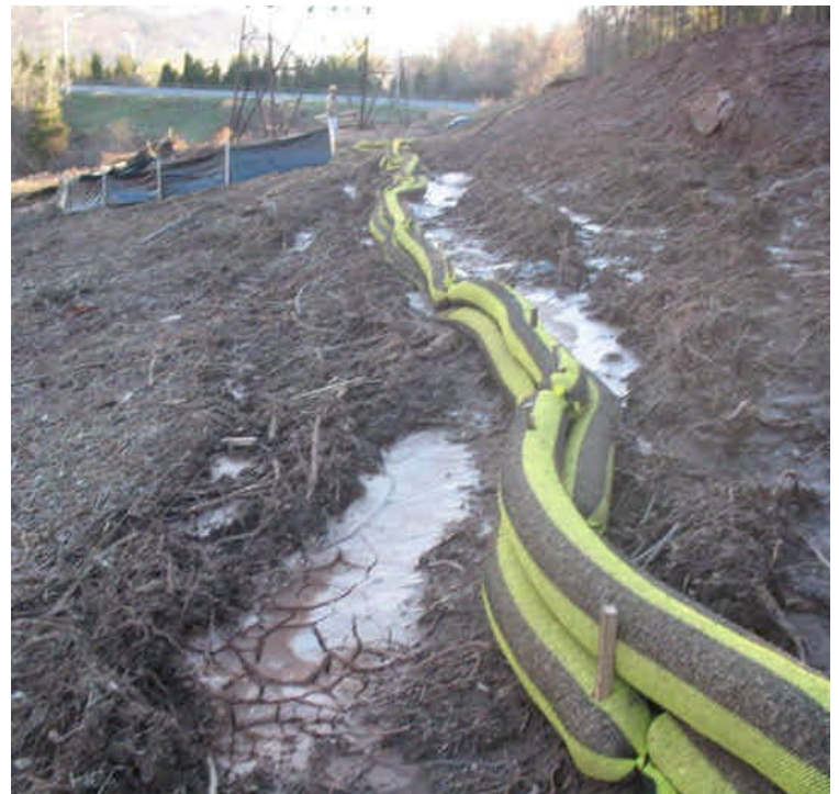
Bio-socks used to trap/filter slurry and sediment from dewatering efforts at Black Pond
