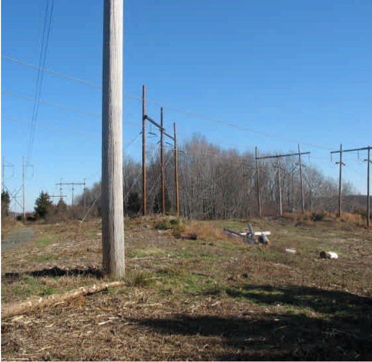
Pole installation complete at Oxbow Junction.
