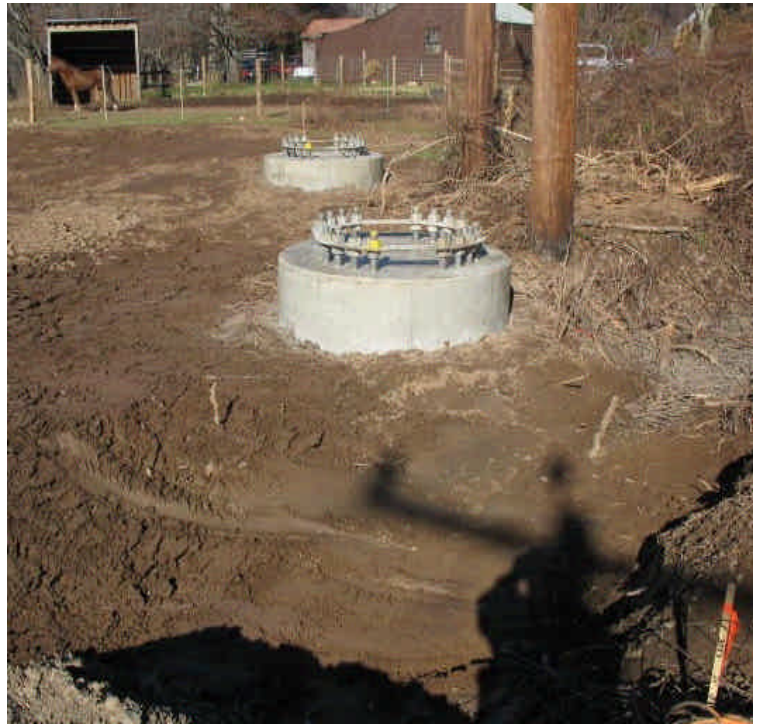
Newly installed foundations off Rt 17 with slurry removal area.
