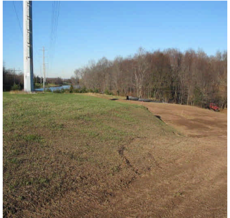
Grass growth noted along cleared slopes north of Beseck SS.
