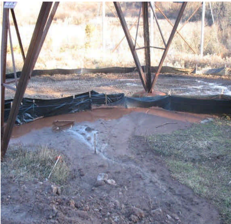
Silt fence/haybale barrier along the access road adjacent to Black Pond, used for dewatering slurry.
