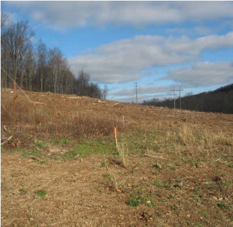
Cleared area north of Beseck SS, prepared for foundation installation.
