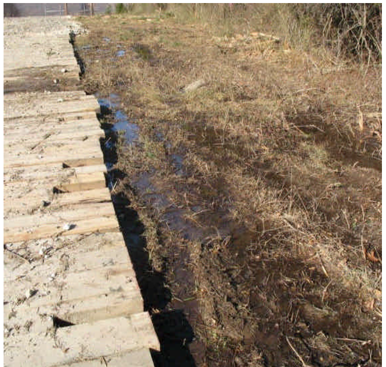
Non-jurisdictional wetland crossing area in the access ROW off Haddam Quarter Rd. Mats are in place and clean water was leaving the site.
