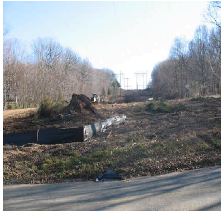
Silt fence installation, clearing and grading off Arbutus Street.
