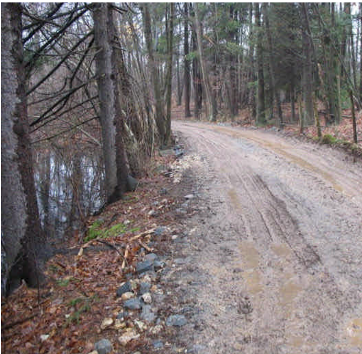
Add erosion controls between the new access road and the pond off Haddam Quarter Rd. to prevent sedimentation.
