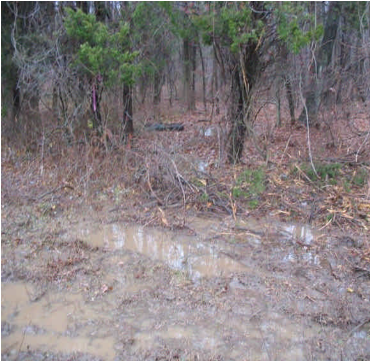
Turbid run-off was noted flowing off site from the wetland crossing off Haddam Quarter Rd. It filters naturally through the vegetation but controls could be installed.
