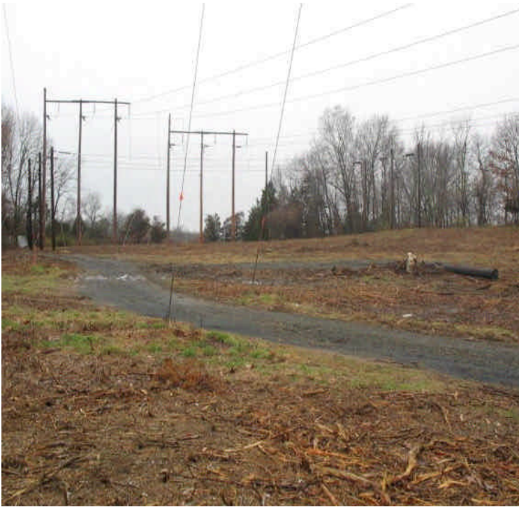
Pole installation complete at Oxbow Junction.
