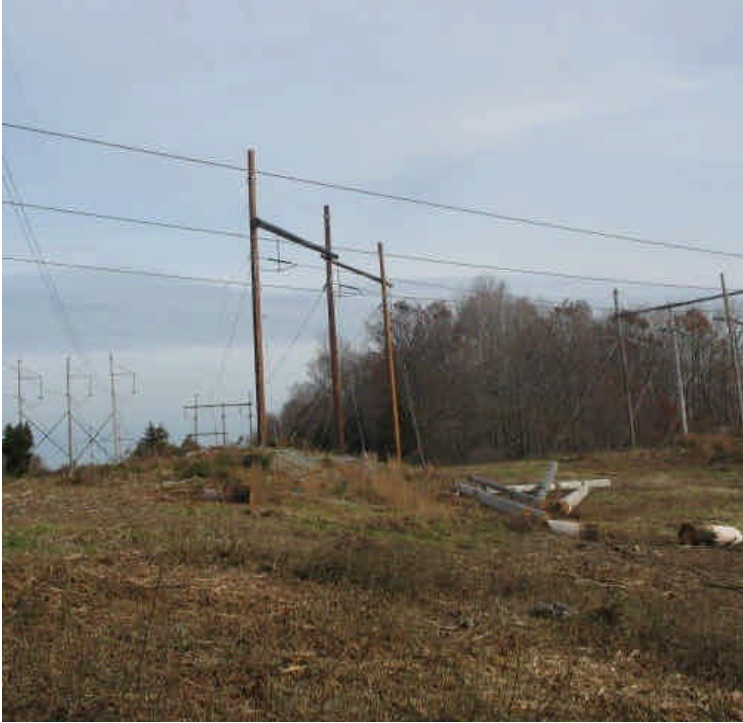
Pole installation complete at Oxbow Junction.
