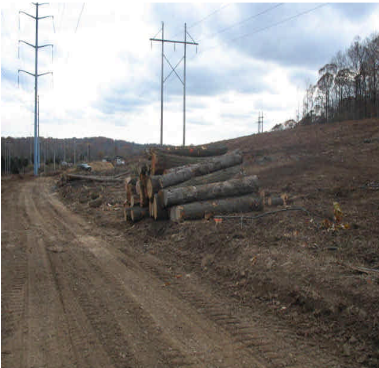
Cleared area north of Beseck SS.
