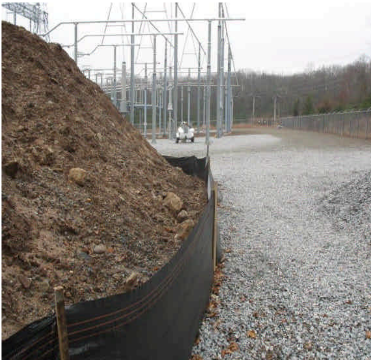
The remaining soil stockpile is surrounded by silt fence and stone.
