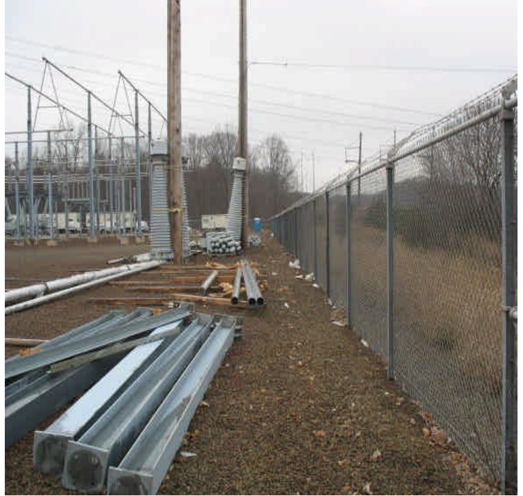
View of the perimeter of the yard. The site is stable and soil disturbing work is now complete.
