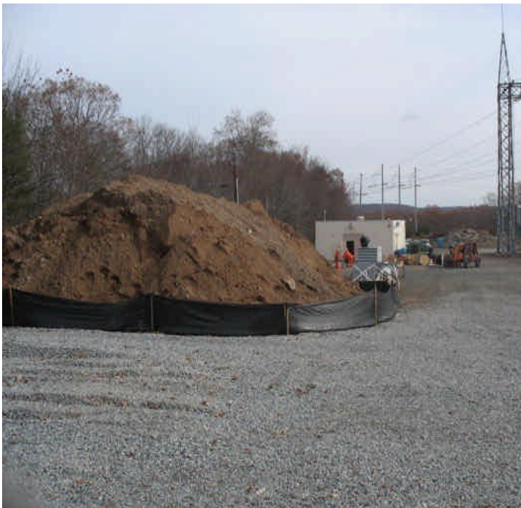
The remaining soil stockpile is surrounded by silt fence.
