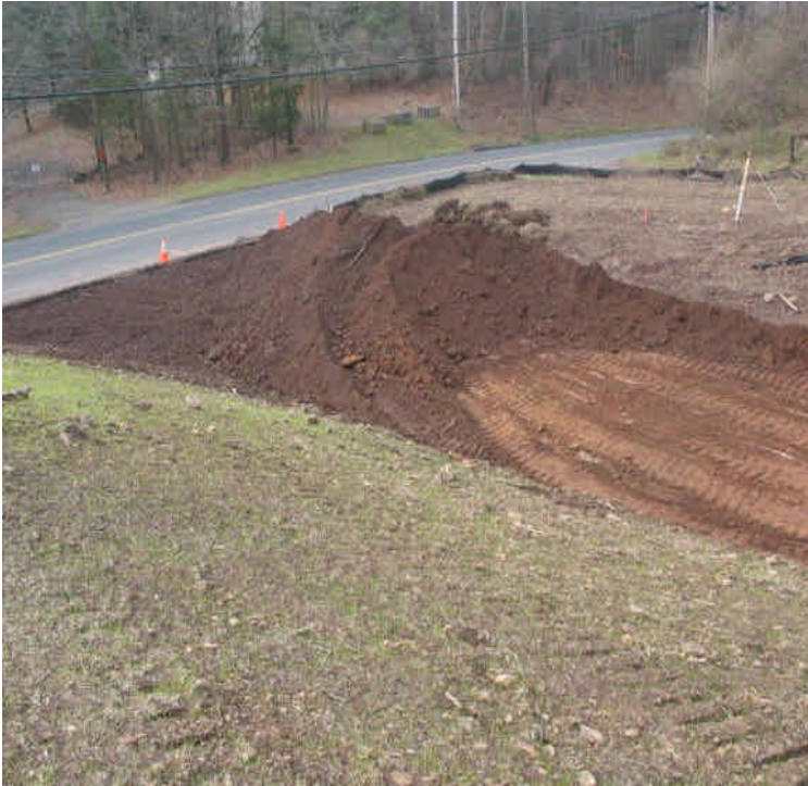
New entrance off Carpenter Lane is being filled and graded.
