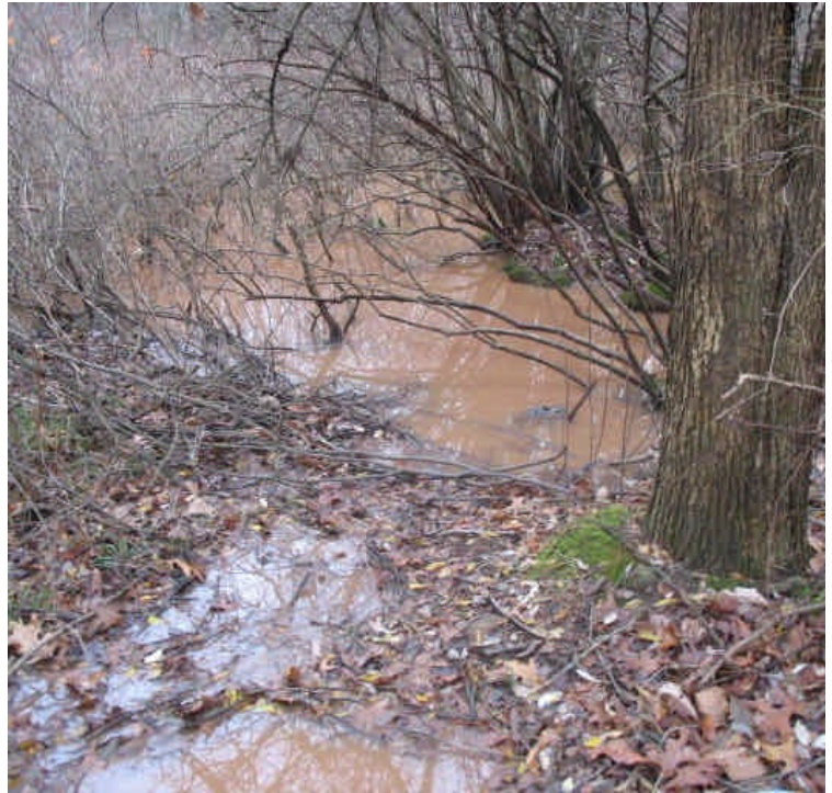
The turbid water had flowed through the haybale barrier and was observed in the wetlands. When this settles out, evaluate whether sediment removal is necessary.
