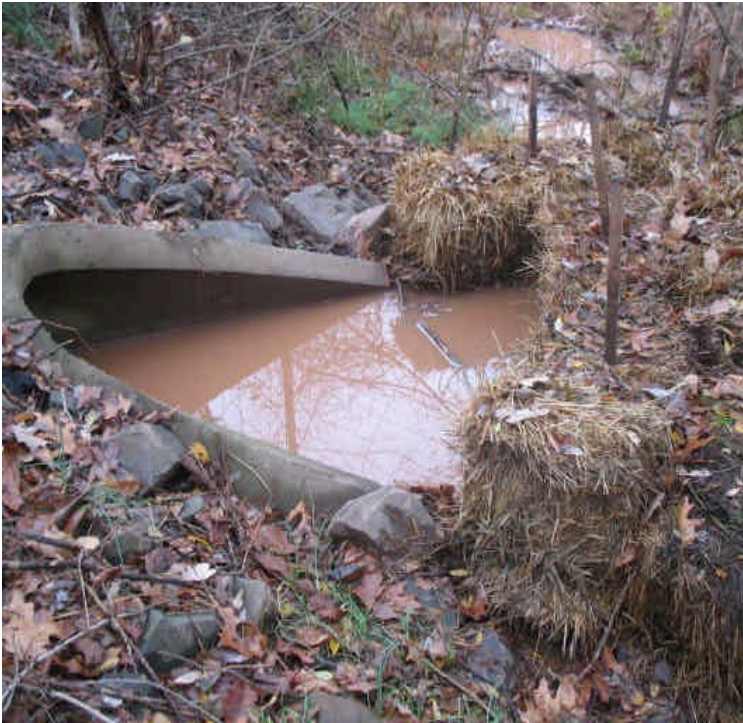
Following several large rain events, turbid run-off was again reaching the storm drain outlet across Carpenter Lane. This issue needs immediate attention again to determine the source and control it.
