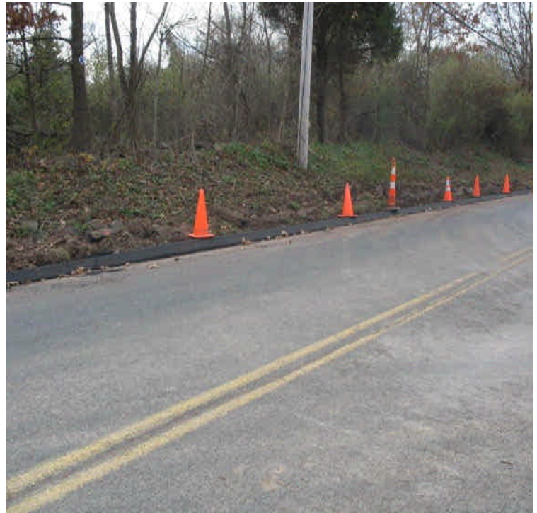
Asphalt curbing has been replaced across Carpenter Lane.
