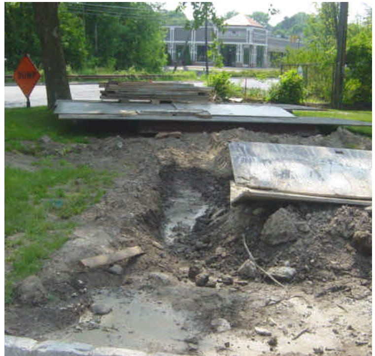
Photo of trenching activities at sta. #365.
