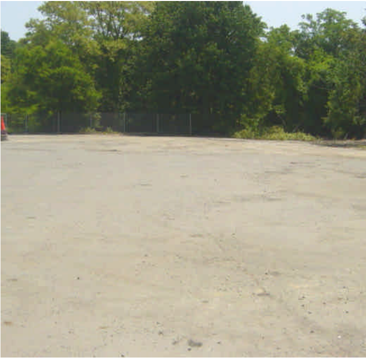
Most of the stored items within the Imperial Ave. lay-down yard have been removed as the yard is being demobilized.
