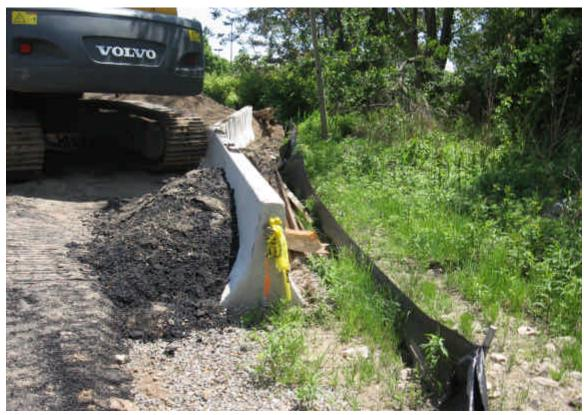
The majority of the compromised silt fence within the King's Highway lay-down yard has been re-established. The portion of the fence in the foreground of the photo required additional reinforcement when feasible.
