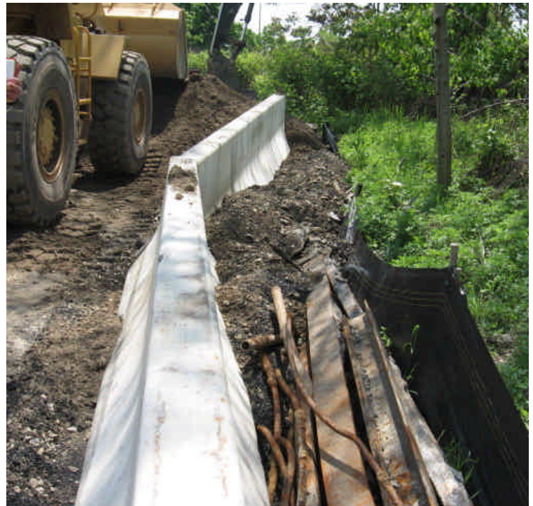
Both photos were taken within the King's Highway lay-down yard. Left: Accumulated slurry remains adjacent to the disposal soil pile. Right: Material is still overwhelming the silt fence perimeter control within the yard. Pull the soil back and restore the controls. However, resource areas are not located adjacent to this area.
