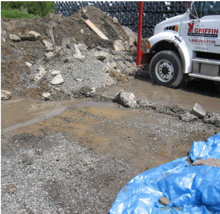
Both photos were taken within the King's Highway lay-down yard. Left: Accumulated slurry remains adjacent to the disposal soil pile. Right: Material is still overwhelming the silt fence perimeter control within the yard. Pull the soil back and restore the controls. However, resource areas are not located adjacent to this area.
