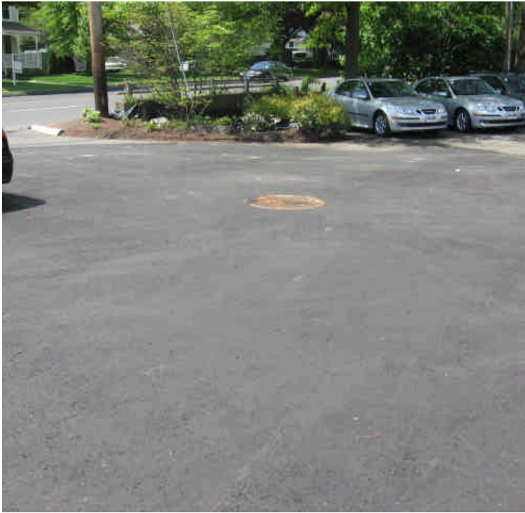
Photo of vault #13 where construction is complete and the area was repaved. Erosion controls remain in place for future trenching activities in the area.
