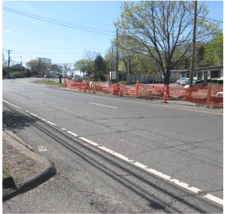
Trench from sta. #312 to #316 is covered with plates, connecting to vault #19.
