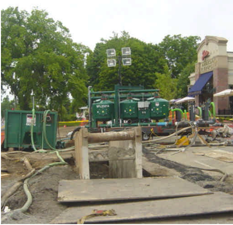
Open trench and ongoing dewatering activities near vault #36.
