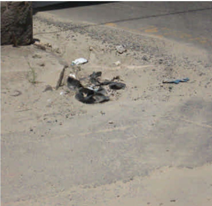
Catch basin location on the corner of Railroad and Myrtle Ave. Accumulated sediment is not project related, but a result of regular tracking attributed to a storage yard for a project not covered under this D&M plan.
