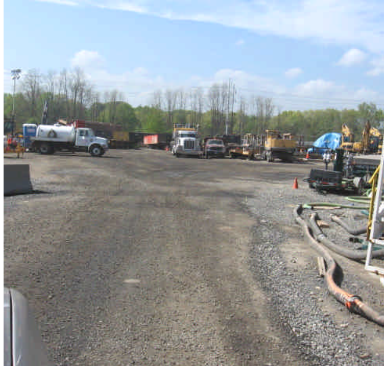
Calcium chloride has been applied to the yard in an effort to prevent dust migration proactively.
