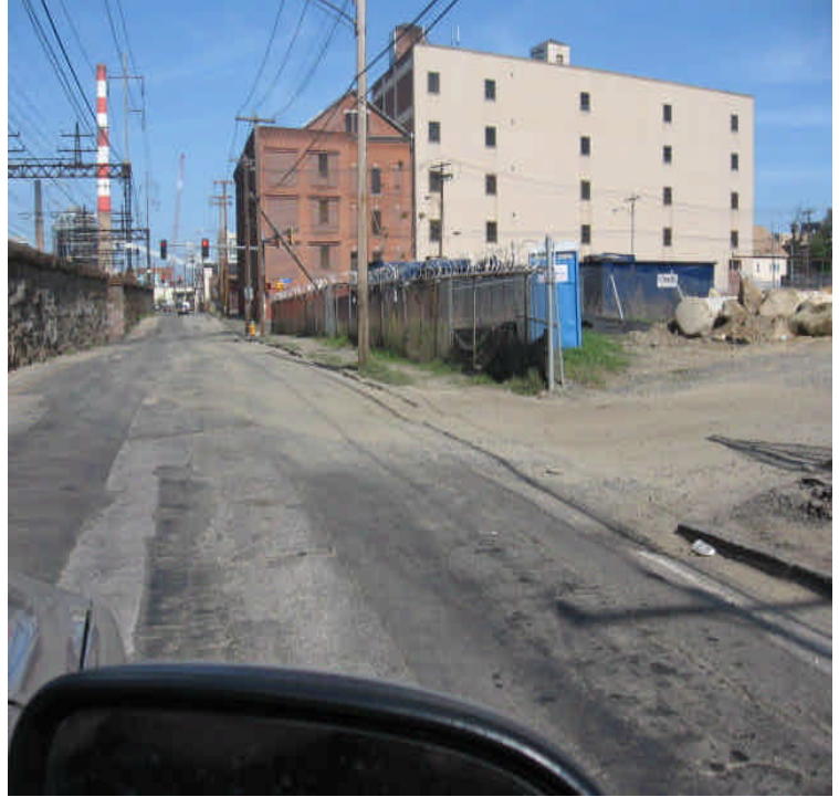
Photo of Railroad Ave. at its intersection with Myrtle Ave. Sediment tracking is regularly noted at this location but is due to a storage yard for a project not covered under this D&M plan.
