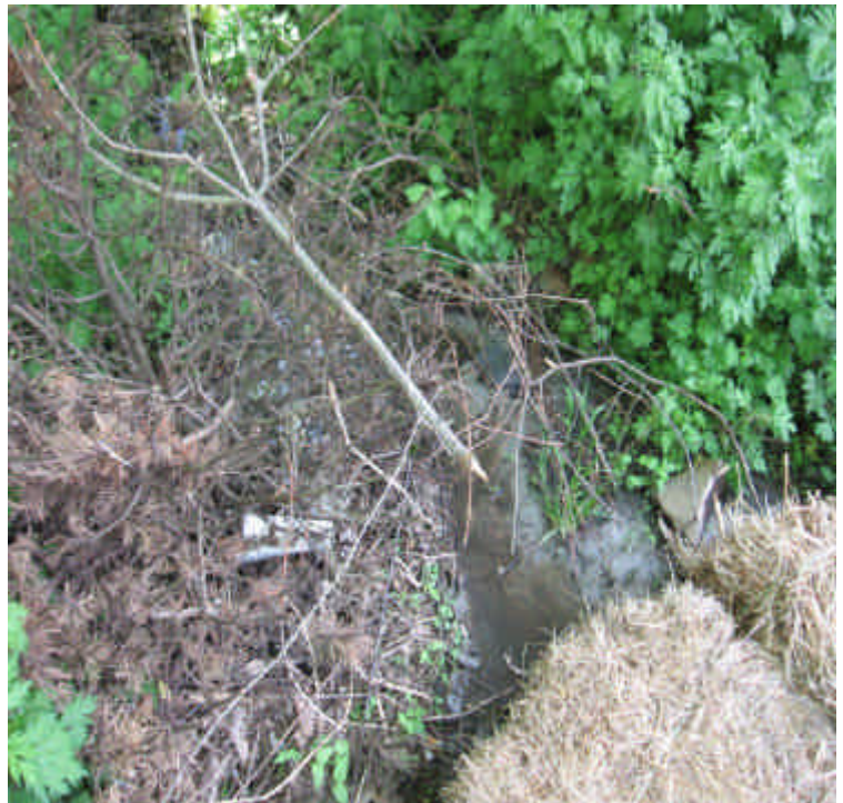
Left: The flowable fill film or slurry has accumulated over a large surface area of the adjacent pavement, with the majority contained within the erosion control barriers. Right: A portion of the flowable fill has migrated just beyond the erosion control barrier in one location and was noted for approximately 5-feet along a drainage channel leading to an adjacent brook. No fill has reached the brook at this time. Contractor was aware of the clean-up requirements at the time of the site visit.
