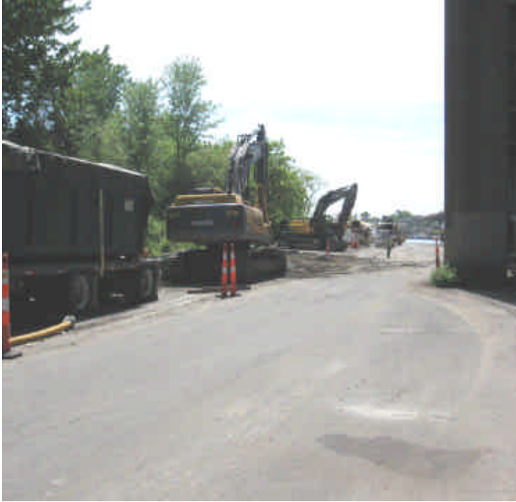
Photo shows an overview of the construction area.
