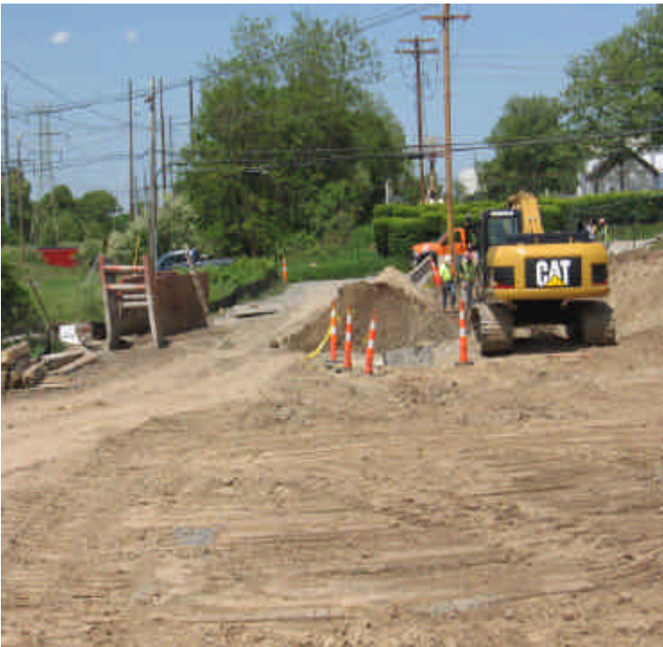
Construction/trenching activities continue at station #1080.
