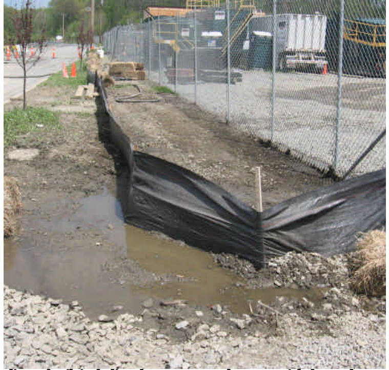
Both photos of the Milford lay-down yard. Left: Equipment removing disposal soil, including the concrete washout material observed here during last week's inspection. Right: Efforts were made to remove sediment that had accumulated adjacent to the erosion controls at the entrance. Seed and mulch may be necessary to stabilize the exposed soil and reduce future run-off to the catch basin.
