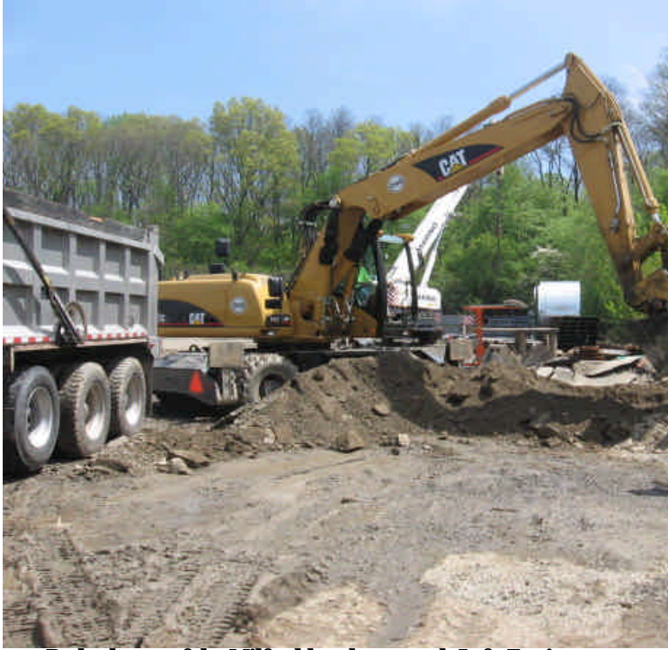
Both photos of the Milford lay-down yard. Left: Equipment removing disposal soil, including the concrete washout material observed here during last week's inspection. Right: Efforts were made to remove sediment that had accumulated adjacent to the erosion controls at the entrance. Seed and mulch may be necessary to stabilize the exposed soil and reduce future run-off to the catch basin.
